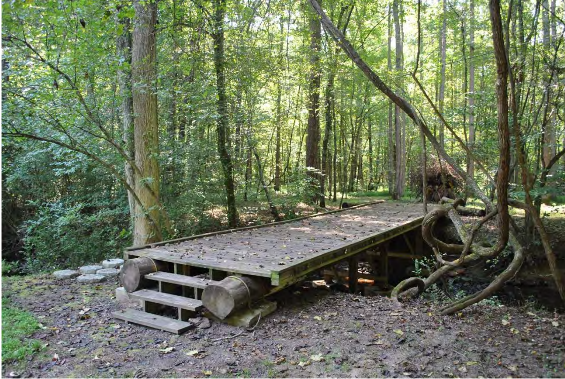
Washington-Ormand Furnace Tract, Modern Foot Bridge Over Long Creek, Looking South.
