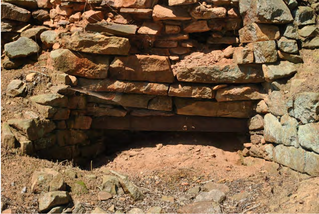
Washington-Ormand Furnace, Fire Opening, Looking West.
